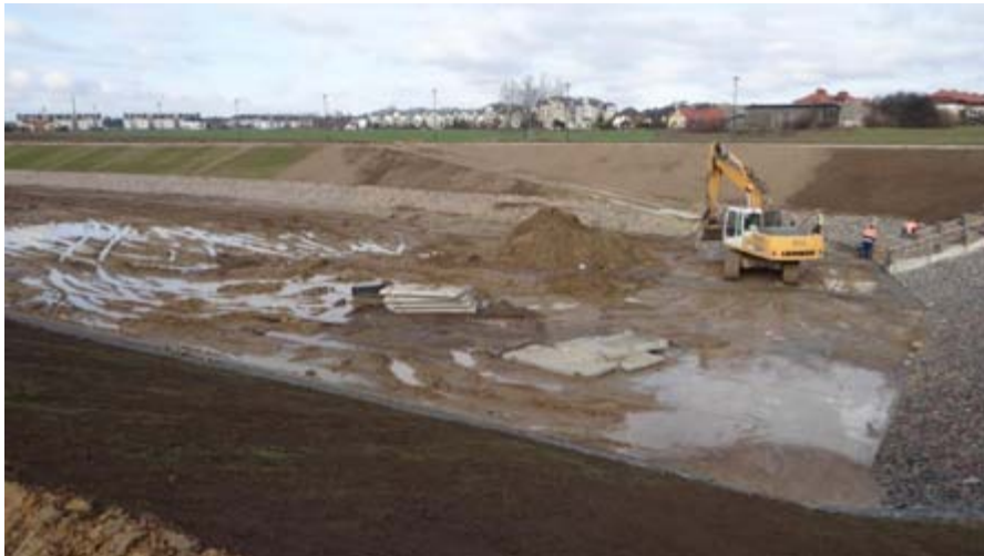
Osowa II reservoir under construction
