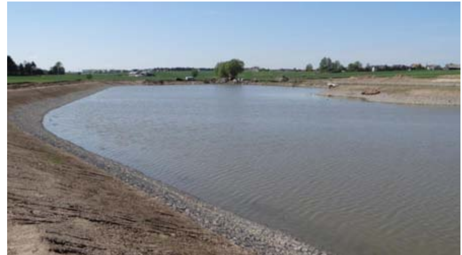
Strzelniczka II reservoir under construction
