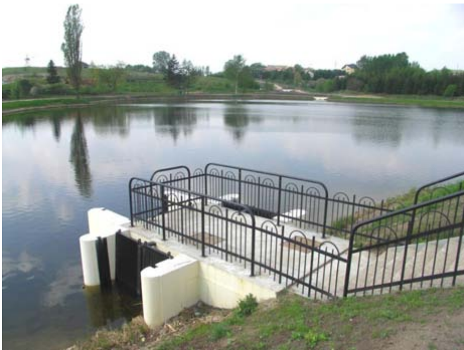
Outlet structure from the reservoir
