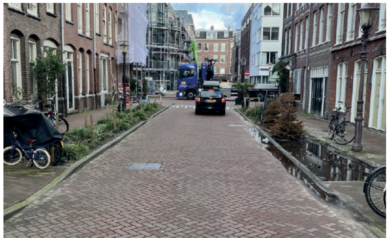
Figure 61: Rain garden on a street in Amsterdam, showing different outcomes using the same stormwater management measure. (Photo credits: author)
