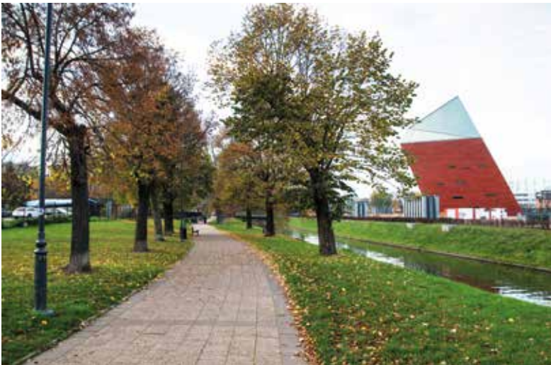
Figure 76: Decommissioned structures along the South bank of river Tagus, Portugal.
