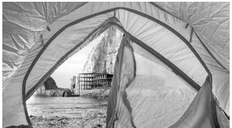
Figure 4: Good Morning Eyesore . Unfinished hotel in Alimuri, demolished on November 30th, 2014, Naples, Italy. (Photo credits: photomontage, S. Antoniadis, 2022).
